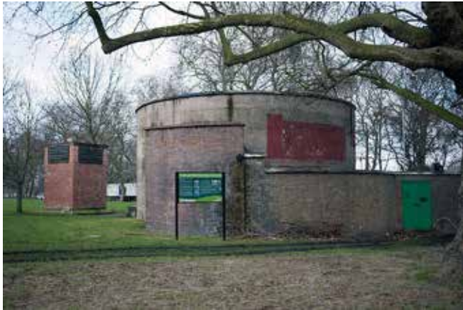
The north entrance on the corner of Clapham Common, opposite Clapham South tube station. The green interpretation installed by Lambeth Council, in co-operation with Sub Brit is prominent. Photo Konstantin Binder
